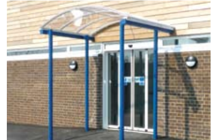
Entrance door canopy
